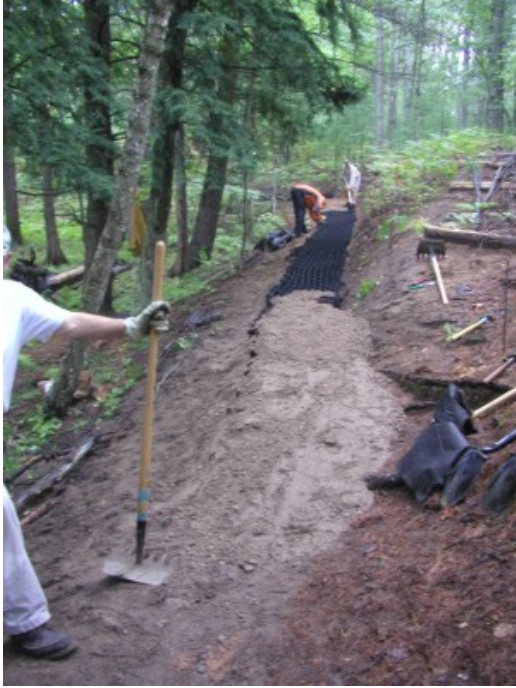
Volunteers install GeoWeb material to stabilize and harden the trail surface.
