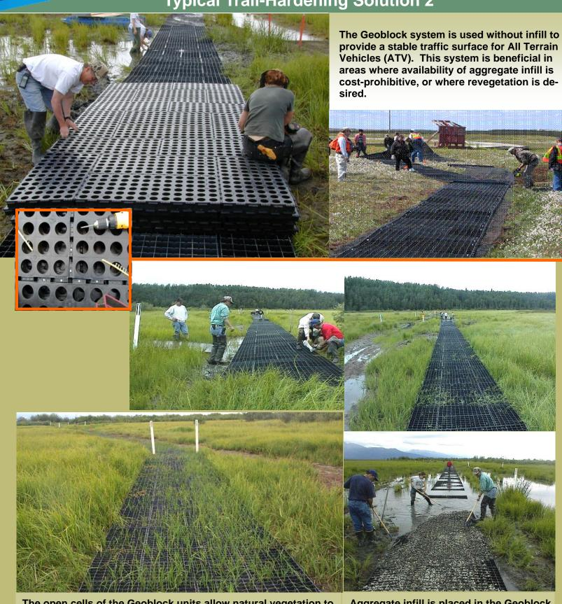
The open cells of the Geoblock units allow natural vegetation to be established through the units.
