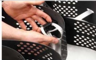
**STEP 3:** Pull the tendon up and over the post of the ATRA Tendon Clip.
