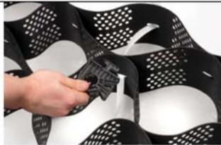
**STEP 1:** Locate the cells where the ATRA Tendon Clips will be installed. Insert the locking member of the ATRA Tendon Clip through the slot in the GEOWEB cell wall. Turn the clip 90 degrees to lock.
