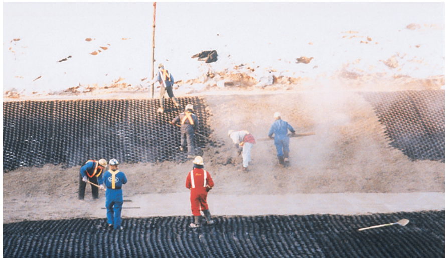
Concrete infill is placed in the cells and raked flush with the top of the Geoweb cells.
