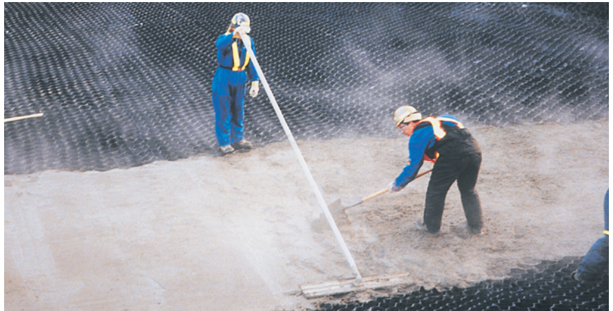
Concrete infill is placed in the cells and raked flush with the top of the Geoweb cells.
