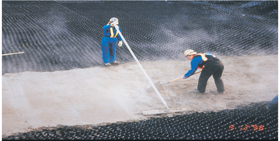
Geoweb sections with two polyethylene-coated tendons per cell and load-transfer clips every four cells are suspended over the liner.
