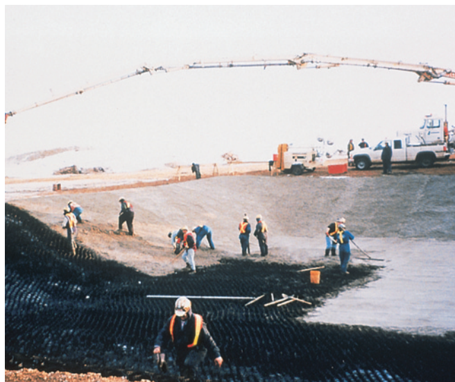
A concrete pump truck is used to place infill in the Geoweb sections.
