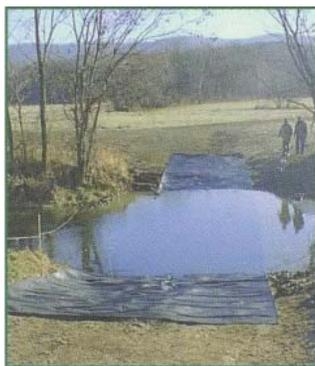
Once the sections were all filled, additional stone was brought in to finish the approaches. The backhoe was used to level and compact the infill. Crushed limestone was used in the stream and local crushed shale for the approaches.
