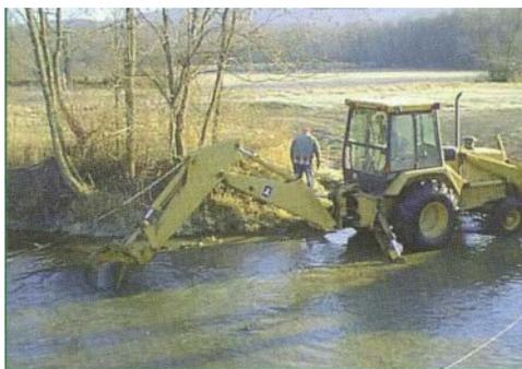
Anchors were evenly spaced and fastened over the tendons within the Geoweb sections to provide security against the stream's up-lift forces. During anchoring, the backhoe dropped crushed stone over the staked Geoweb sections. Equipment can be driven on the system as soon as the Geoweb cells are completely filled.
