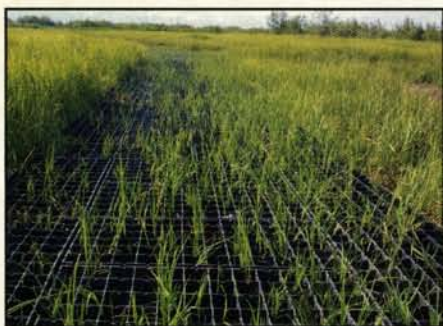
Open grid cell allows for vegetation re-growth.
