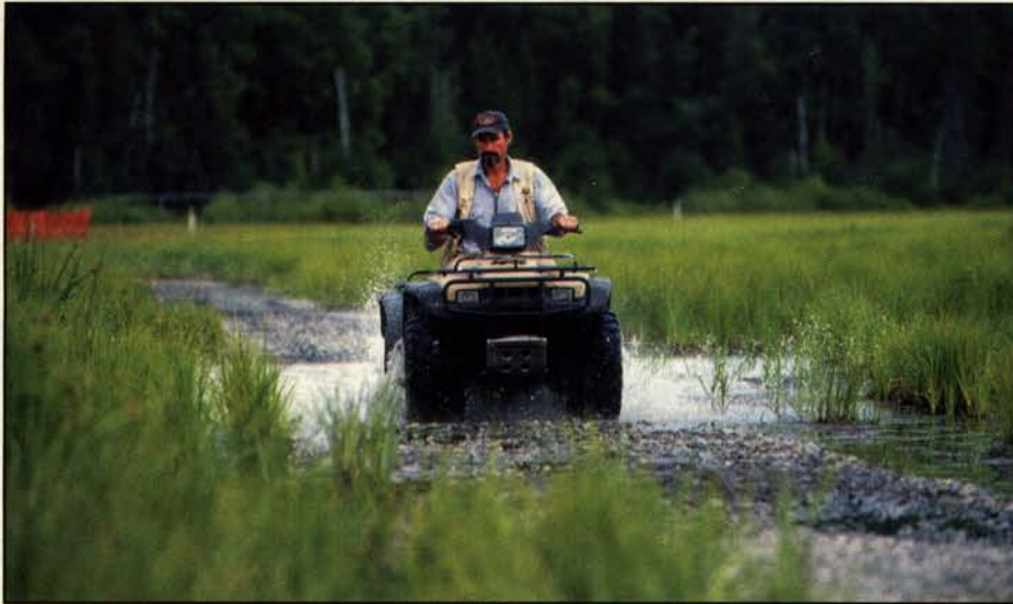
Kevin Meyer, a specialist with the NPS Rivers and Trails Program traverses a newly installed section of hardened trail at the Palmer Hay Flats. Photo credit: Erik Hill, Anchorage Daily News
