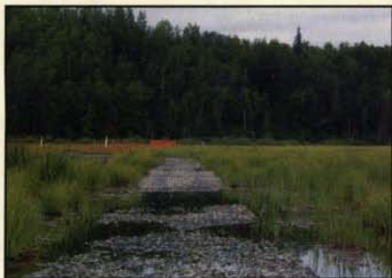
Gravel ballast is used at pond crossings.
