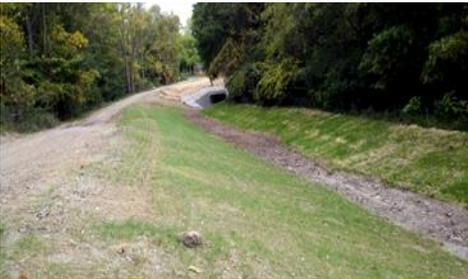
With an overlying TRM, the GEOWEB confinement system stabilizes topsoil infill to resist continuous low-flow channels and high-flow intermittent channels.
