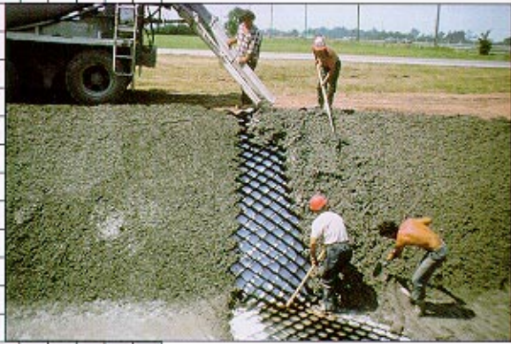
Concrete was poured into the upper Geoweb cells and raked into lower cells.
