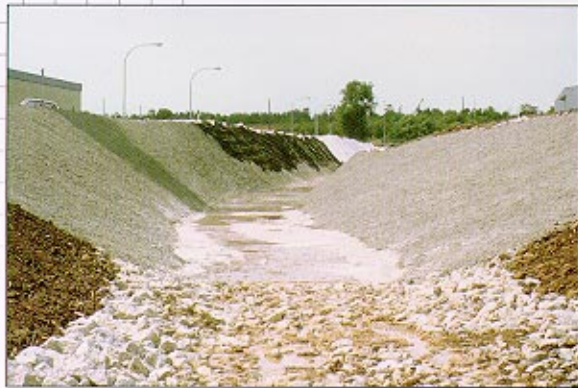
Finished concrete Geoweb channel liner.
