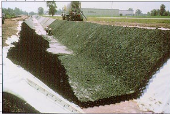
A four man crew placed 1486 square meters of concrete per day.
