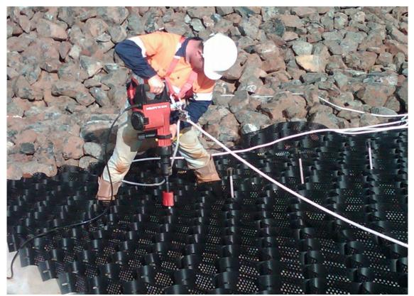
5 Makes Secure Connection with GEOWEB® Cell Walls
