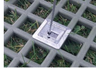
Figure 8. Set Gripple into GeoRunner Panel Opening
