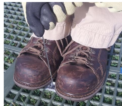
Figure 9. Tighten Gripple to Secure GeoRunner to Ground
