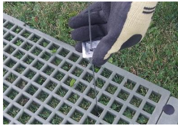
Figure 7. Install Gripple
