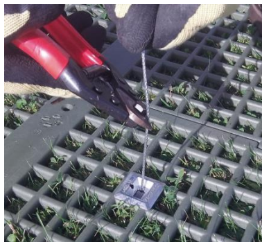
Figure 10. Cut the Cable to Loop the Trailing End
