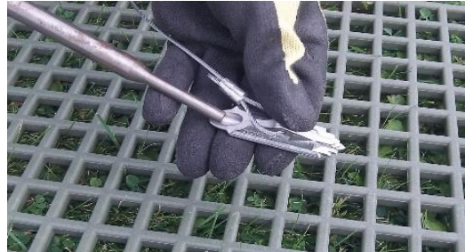
Figure 4. Install Anchor
