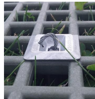
Figure 11. Loop Cable Back in the Gripple
