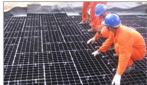
Figure 15: Connecting GEOTERRA Units
