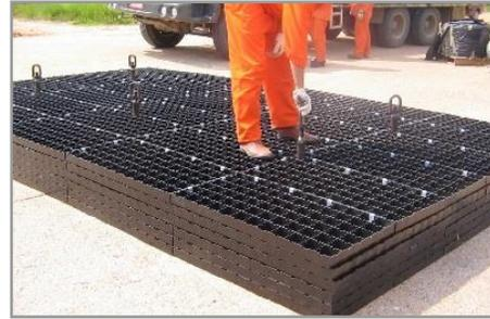
**Figure 28: Assembling GEOTERRA Mats (Side-by-Side Pattern)**
