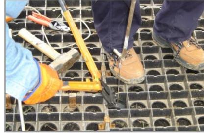
**Figure 34: Crimping the Cable Stop**
