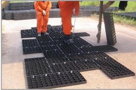
**Figure 27: Assembling GEOTERRA Mats (Herringbone Pattern)**
