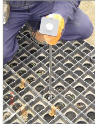
Figure 31: Installing the Earth Anchor
