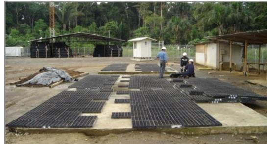
**Figure 30: Connecting Pre-Assembled GEOTERRA Mats**
