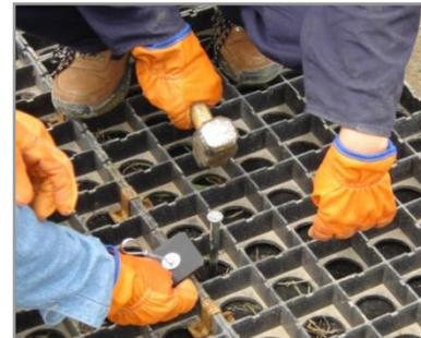
Figure 32: Driving the Anchor Head
