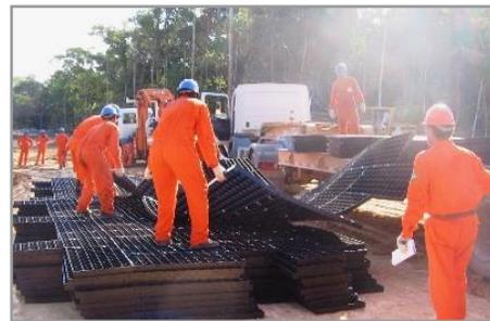
Figure 26: Transporting Pre-Assembled Mats from Off-Site
