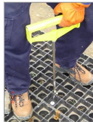
Figure 33: Setting the Earth Anchor
