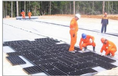
**Figure 29: Placing GEOTERRA Mats Over Geotextile Layer**
