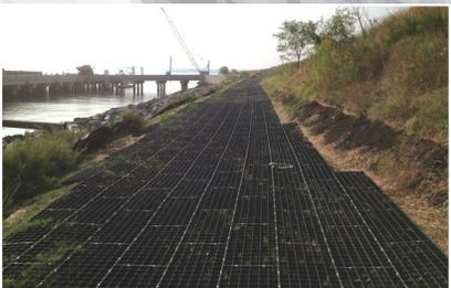
GEOTERRA Mats installed for a 15 ft. wide x 3000 ft. long roadway allow site access in an environmentally sensitive area with minimal impact.
