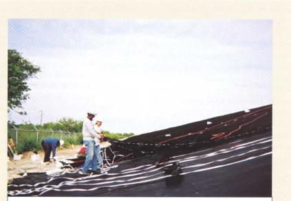
**Photo 2.** Installation of the geocellular system over geotextile and geomembrane.
