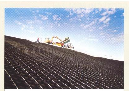
*Photo 3*. The slope during its final stage: aggregate is unloaded and raked into the cells.
