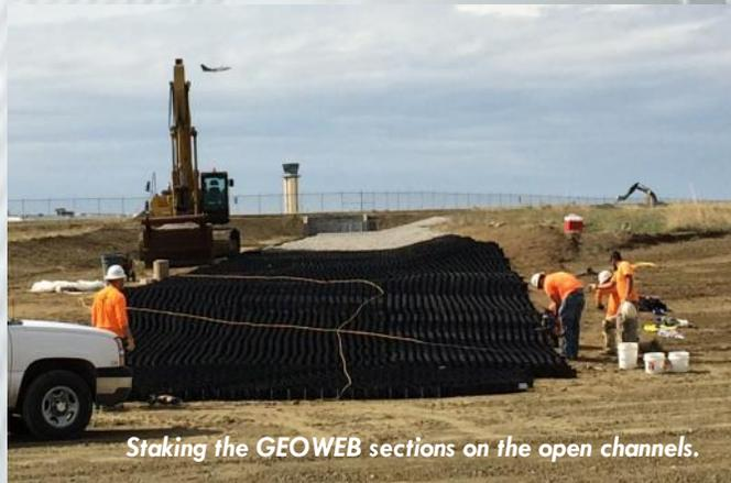
*Staking the GEOWEB sections on the open channels.*
