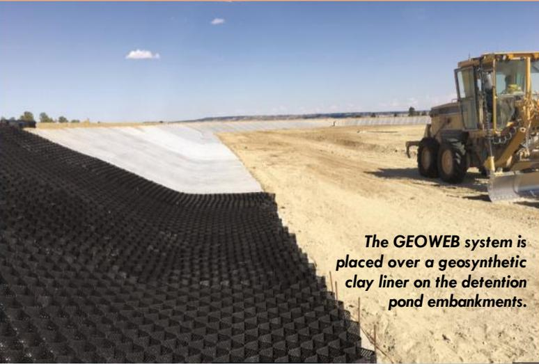
*The GEOWEB system is placed over a geosynthetic clay liner on the detention pond embankments.*
