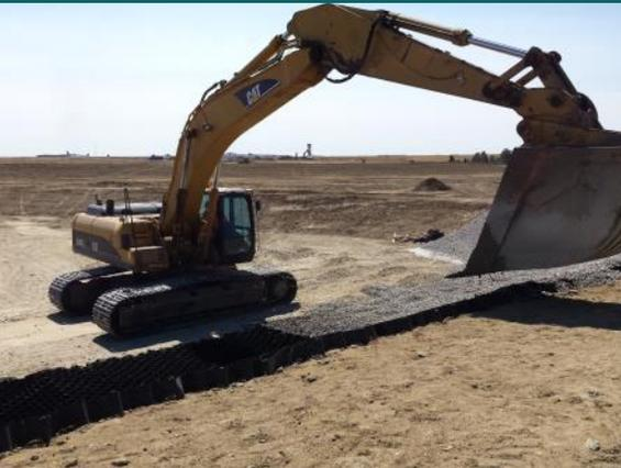
*Infilling GEOWEB sections with aggregate for storm water detention pond perimeter protection.*
