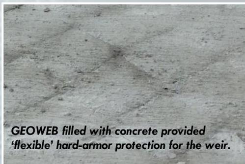
*GEOWEB filled with concrete provided 'flexible' hard-armor protection for the weir.*
