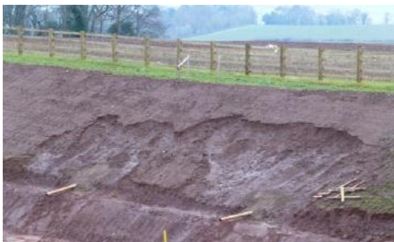
Cut slope prior to stabilization
