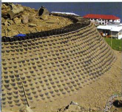
The protection system's outer walls, when filled with soil provided an environment to support native vegetation.
