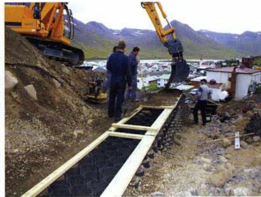
The protection system's outer walls, when filled with soil provided an environment to support native vegetation.
