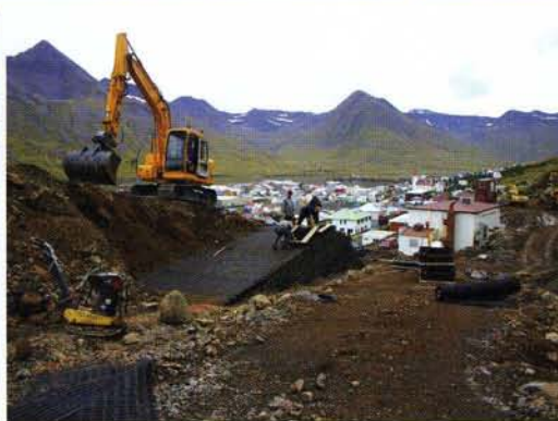
The protection system's outer walls, when filled with soil provided an environment to support native vegetation.
