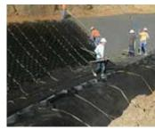
Presto's ATRA Tendon Clips make a secure connection with the GEOWEB cell wall for transferring loads from the tendon to the cell wall.
