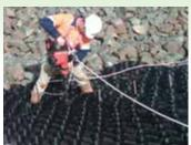
Presto's ATRA Anchors make a secure connection with the GEOWEB cell wall and are fast and easy to drive with ATRA drivers.
