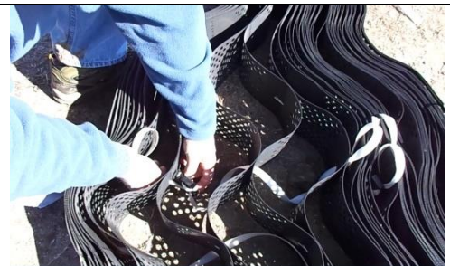
Figure 10 Preassembling ATRA Tendon Clips
