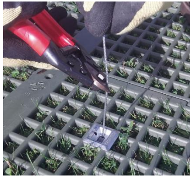
Figure 10. Cut the Cable to Loop the Trailing End
