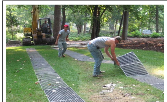
Figure 1. GeoRunner Panel Installation
