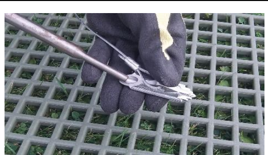
Figure 4. Install Anchor
