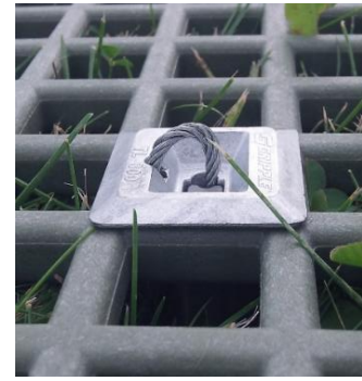
Figure 11. Loop Cable Back in the Gripper
