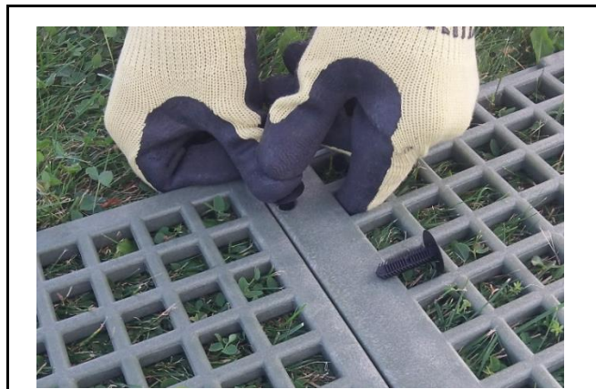
Figure 2. Install Rivets
