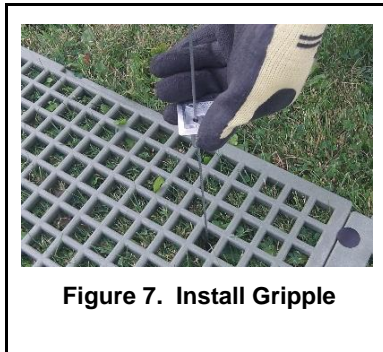
Figure 8. Set Gripple into GeoRunner Panel Opening
