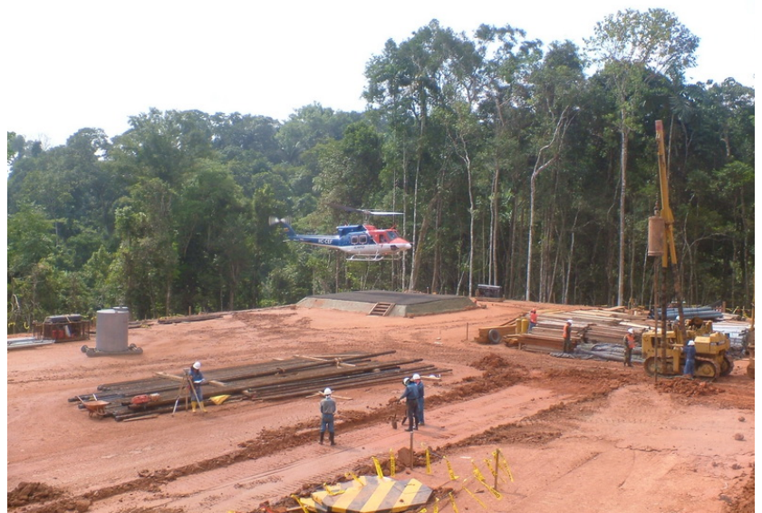
The GeoTerra system weighs approximately 9 kg per square meter. A helipad this size can easily be transported in two preassembled sections.
