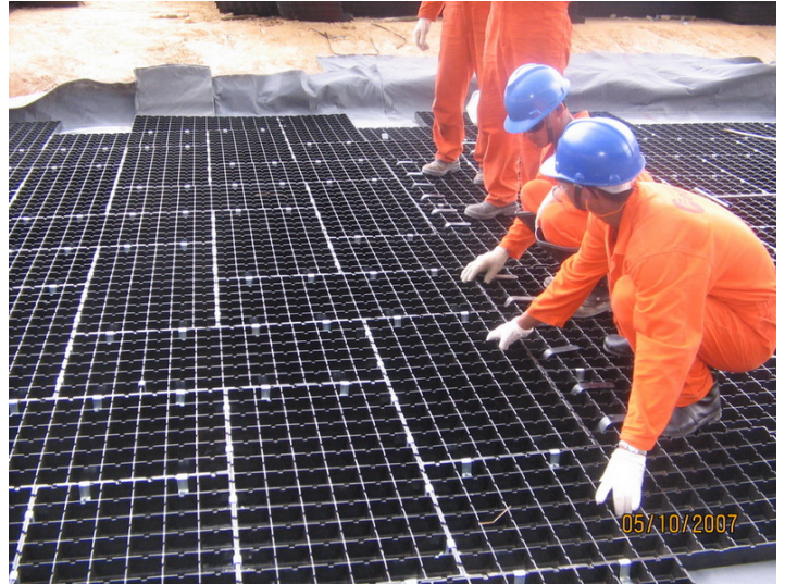
The helipad system is assembled using 0.5 m x 1.0 m individual GeoTerra units that are typically pre-assembled into larger mats either on or off site, flown into the site and assembled to the dimension of the landing area.
