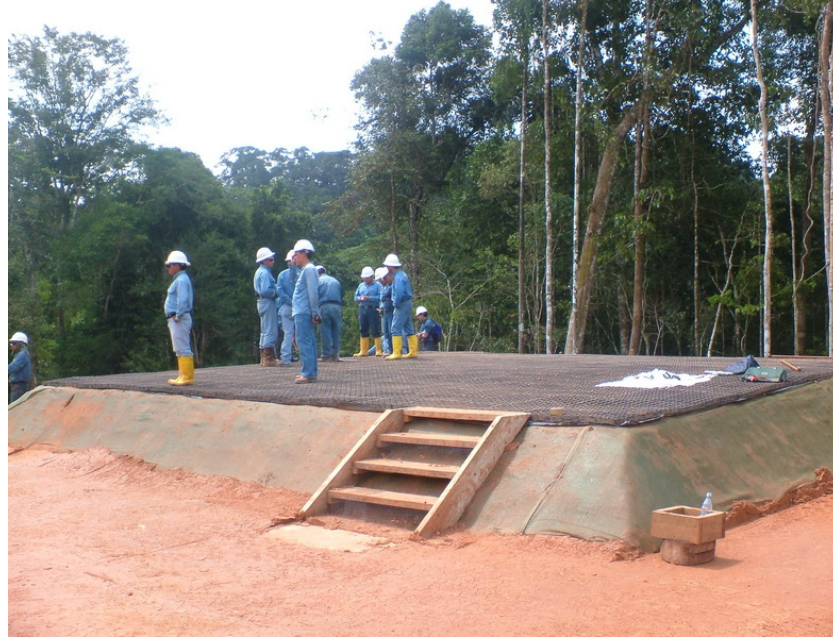
Typical landing / takeoff areas for personnel may be as small as 5 m x 5 m but will always be dependent on the size of the helicopter.
