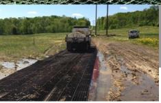
GEOTERRA Mats can be configured to fit any site requirement. GEOTERRA sections are typically placed over a high strength geotextile.
