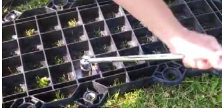
Figure 21: Auger Anchor Install with Breaker Bar
