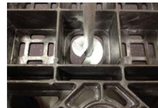
Figure 20: Insert Auger Anchor through Open Cell
