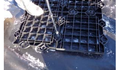
Figure 18: Final Tightening of Nuts
