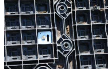
Figure 23: Installed Auger Anchor
