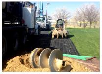
GEOTERRA GTO Mats support heavy drilling equipment across lawn during construction of baseball field lights.
