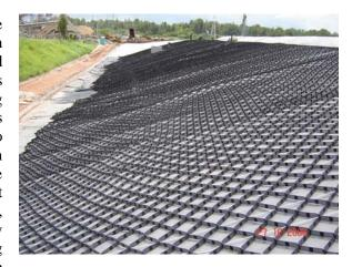
Tendoned Geoweb sections installed and ready for sand infill.
