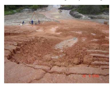
The failed original slope cover viewed from the crest of the slope down.
