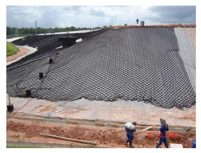
Installation of the perforated Geoweb® sections over the textured geomembrane.
