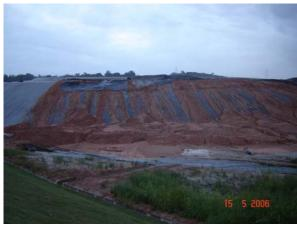
Damaged geotextile resulting from slope failure.
