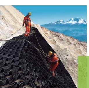
Designed for additional stability by integrating tendons on steeper slopes or when a geomembrane or hard soil/rock surface prevents anchoring with stakes.
