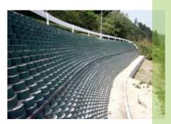
Where vegetation is not desired, GEOWEB walls support aggregate infill or concrete grout.
