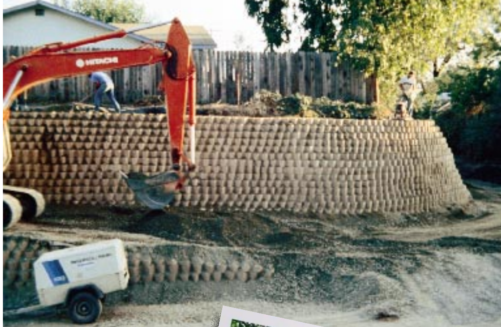
Geoweb gravity wall construction.
