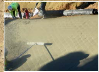
Finishing the concrete surface
