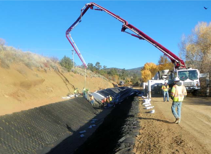
A pump truck is used to install concrete in the GEOWEB sections on the canal slopes. The 3D geocell structure allows a higher slump concrete to be used, facilitating quicker placement by a pump truck, and significantly improving installation time.
