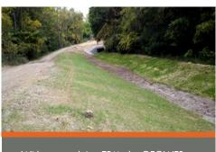
With an overlying TRM, the GEOWEB confinement system stabilizes topsoil infill to resist continuous low-flow channels and high-flow intermittent channels.
