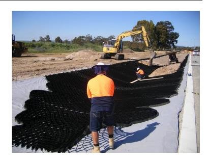
Geofabrics Australasia suggested a new innovative product called **Geoweb®** cellular confinement system. The swale when constructed was 7.0m wide with a 1 in 3 batter slope.
