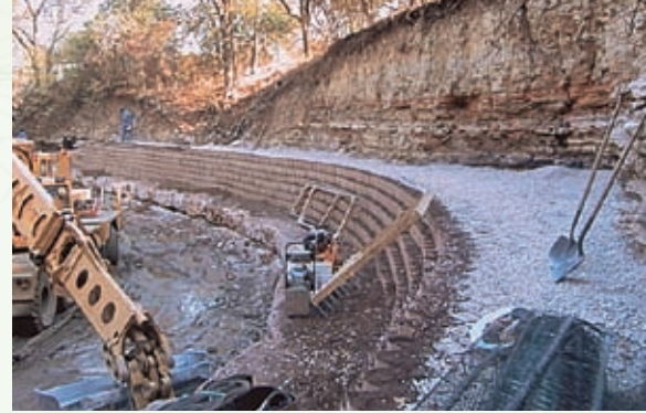
Project photos courtesy Soil Stabilization Products Co.
