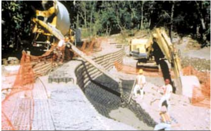
Photo 3: Excavator placing backfill material behind the gravity geocell wall.
