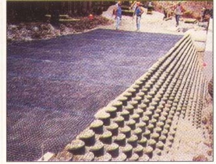
Left: A stretcher-frame is used to keep the Geoweb wall sections open during the infilling process. Center: The fascia is checked for proper elevation, and section alignment and setback before positioning subsequent layers. Right: Biaxial geogrid reinforcement layers are laid between the cellular layers in two-ft lifts or every fourth course.
