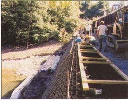
Left: A stretcher-frame is used to keep the Geoweb wall sections open during the infilling process. Center: The fascia is checked for proper elevation, and section alignment and setback before positioning subsequent layers. Right: Biaxial geogrid reinforcement layers are laid between the cellular layers in two-ft lifts or every fourth course.
