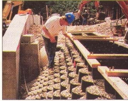
Left: A stretcher-frame is used to keep the Geoweb wall sections open during the infilling process. Center: The fascia is checked for proper elevation, and section alignment and setback before positioning subsequent layers. Right: Biaxial geogrid reinforcement layers are laid between the cellular layers in two-ft lifts or every fourth course.
