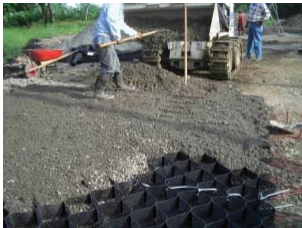
Starting laying the GeoWeb® Service Road
