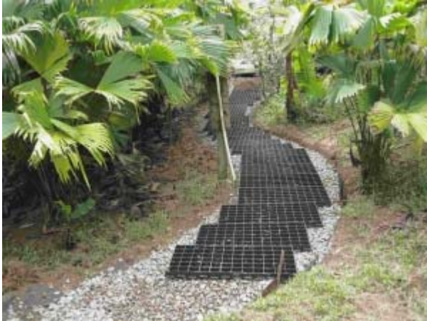
GeoBlock® units laid on a base of course aggregate, and a preview of what a section of GeoBlock looks like.
