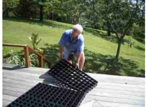
GeoBlock® units laid on a base of course aggregate, and a preview of what a section of GeoBlock looks like.
