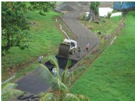
Continued progress of Service Road construction with Geoweb® sections.
