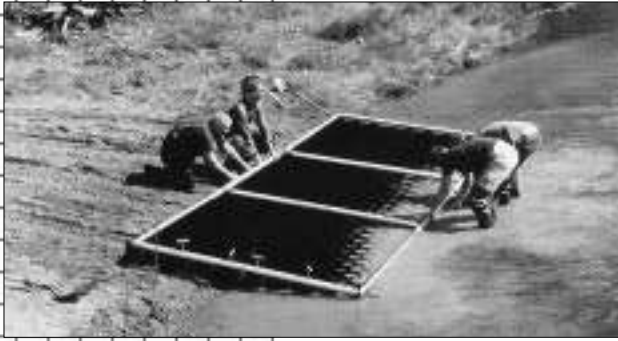
The Presto stretcher frame is used to position GEOWEB sections in the water
