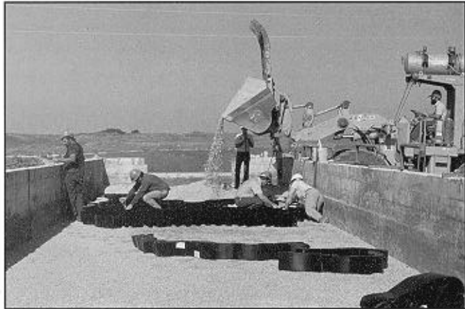
1. The 8 ft x 20 ft x 8 in Geoweb sections were extended, staked and filled with DOT specification filtration sand.
