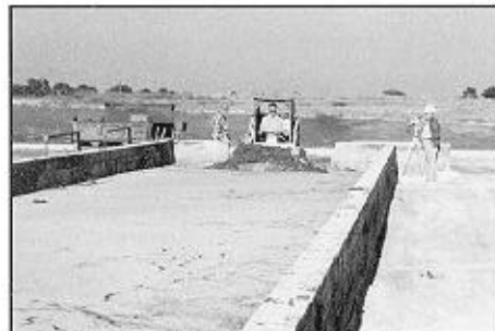
4. A 1,780 sq. ft. drying bed is loaded and cleaned in less than 48 hours.
