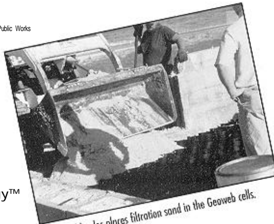
1. The 8 ft x 20 ft x 8 in Geoweb sections were extended, staked and filled with DOT specification filtration sand.
