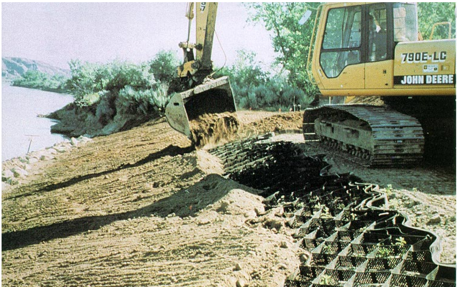
A cellular-confinement system provides structural support to the soil veneer and ensures that a uniform soil thickness is established and maintained on the slope face.
