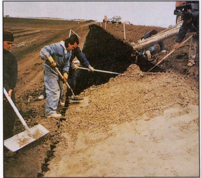
Infilling geocells with concrete.
