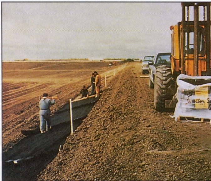
Crews install nonwoven geotextile on the slope before placing geocell panels.
