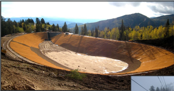
The Geoweb system, typically black, was requested and provided in tan color for this project.
