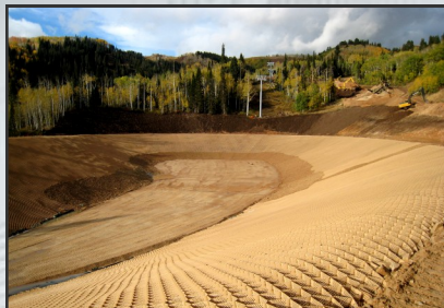
The completed snowmaking pond is protected by a geosynthetic solution including a Bentomat DN, 60 mil textured liner, a 16 oz NW geotextile and the Presto GEOWEB® slope protection system.
