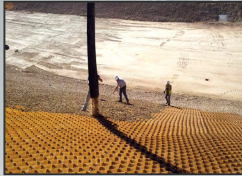
Infilling the Geoweb sections with crushed rock mined on-site.
