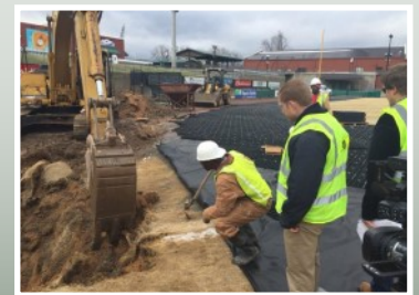
Engineers and officials survey the progress of the sinkhole repair. GEOTERRA Mats are installed to allow heavy vehicle and equipment access in and around the repair site.
