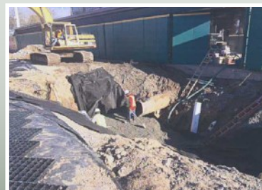
Engineers and officials survey the progress of the sinkhole repair. GEOTERRA Mats are installed to allow heavy vehicle and equipment access in and around the repair site.
