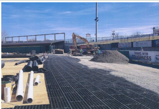
Engineers and officials survey the progress of the sinkhole repair. GEOTERRA Mats are installed to allow heavy vehicle and equipment access in and around the repair site.
