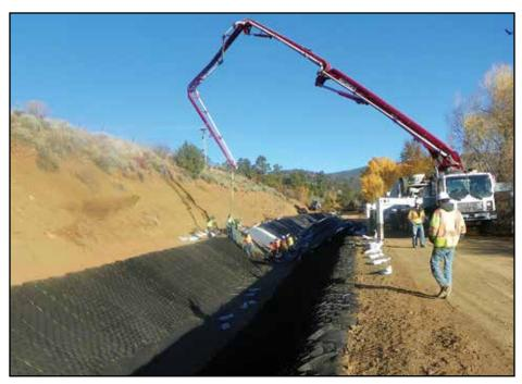
Concrete is pumped into the Geoweb system with a telescoping boom truck.
