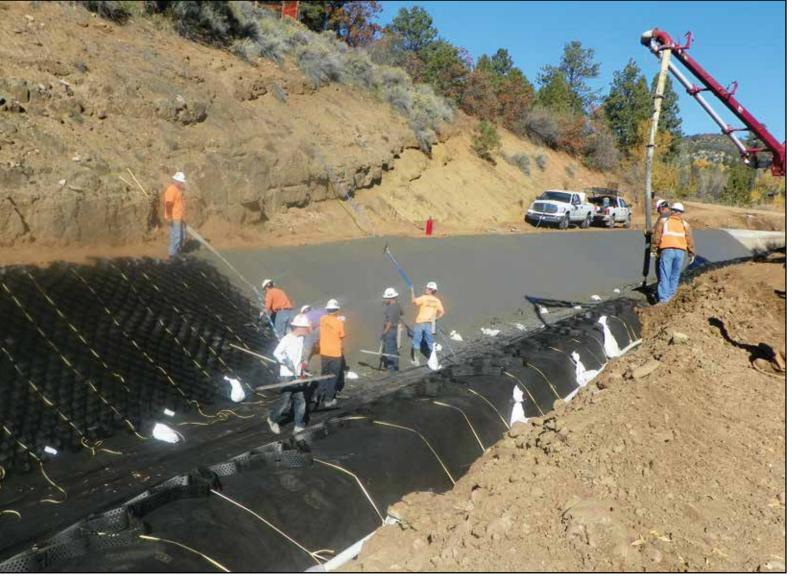
Geoweb sections with a tendon anchoring system and concrete infill protect the impervious channel liner.
