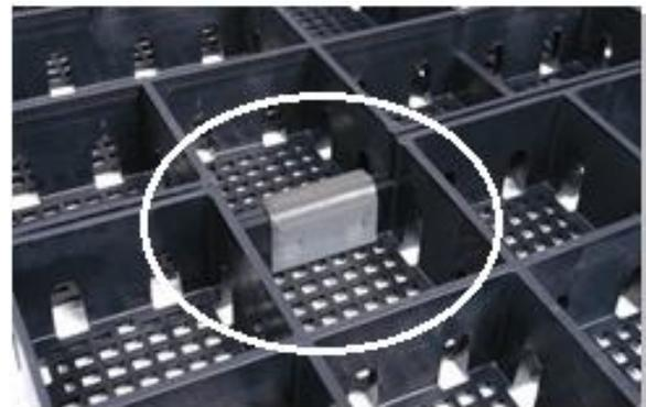
If the U-Clip is not driven down completely, place the driver head over the U-Clip and repeat Step 3.
