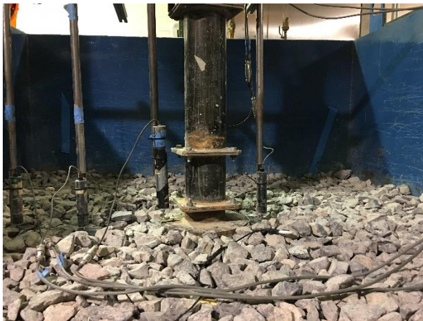
(a) Plate loading test
