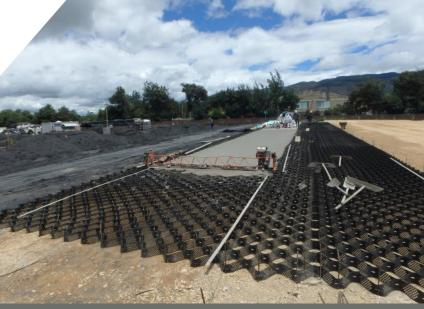
After placement in the GEOWEB cells, the concrete is screeded to remove excess and create a level pavement surface.
