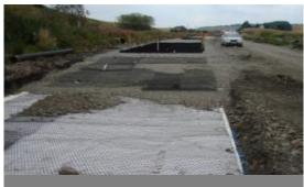
Geotextile & geogrid layers installed prior to GEOWEB 3D aggregate confinement.
