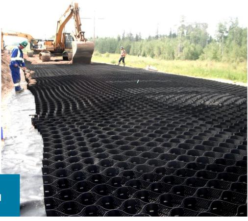
GEOWEB® 3D System and High-Strength Geotextile Combine Forces to Create Upgraded, High-Performing Haul Roads Over Challenging Subgrades.
