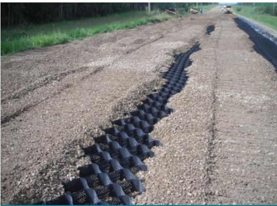
Beneficial Use of Local, Low-Cost Fill
