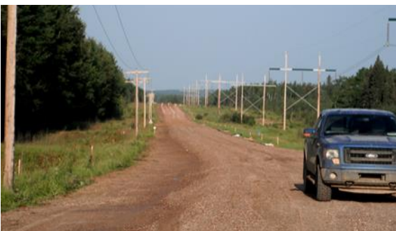
Final Stabilized Haul Road
