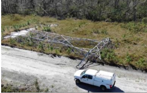
Downed Transmission Towers Duke Energy Photo Credit
