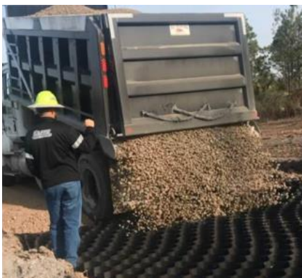
Delivering & Spreading GEOWEB Infill
