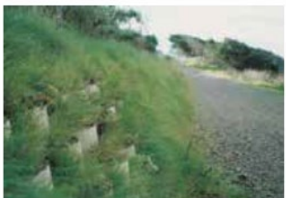
GEOWEB® Slope Protection
