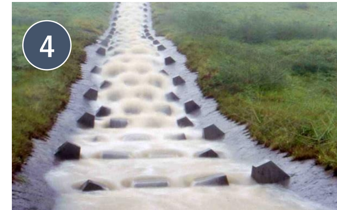
Spillway & Overflow Protection (p. 21-22)
